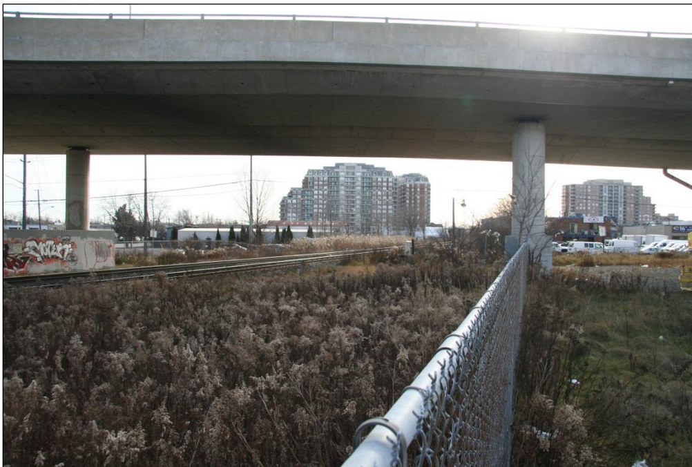
Plate 6: View of 16 th Ave, Facing South (Note Railway, Road, and Building Disturbance)
