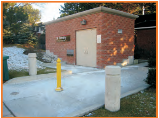
Example of an Emergency Exit Building from Sheppard Subway
