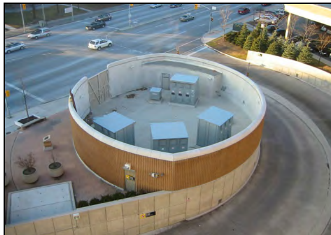
Aerial view of Don Mills Station substation showing substation enclosure
