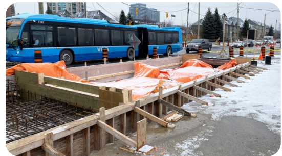
Concrete forms in place for a vivastation
