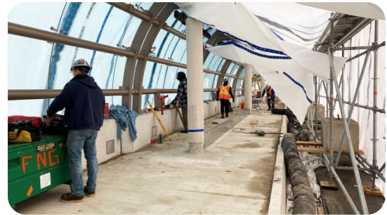
Winter work underway inside a tarp-covered vivastation
