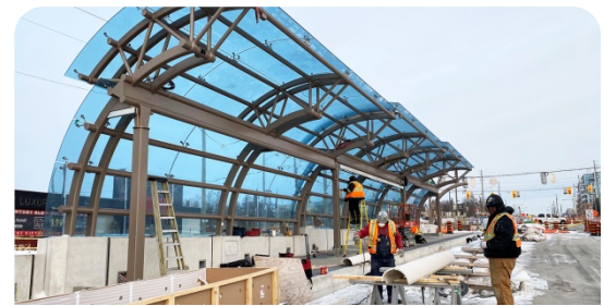
Vivastation canopy glass installed
