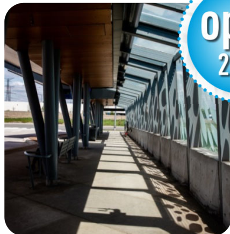
YRT Bus Terminal at Pioneer Village Subway Station
