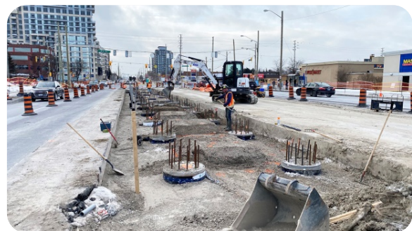
Vivastation foundations underway on Yonge St.
