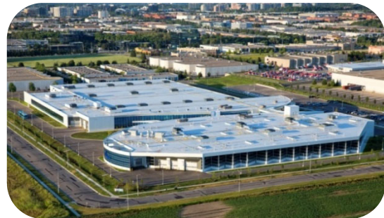
Aerial view of the Operations, Maintenance and Storage Facility
