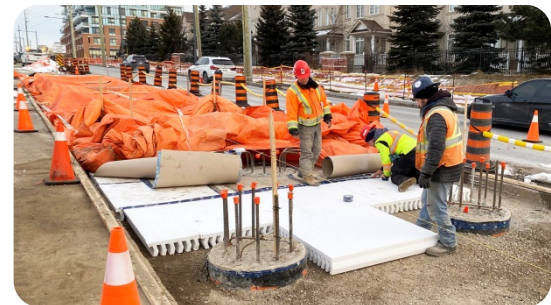
Vivastation foundations underway
