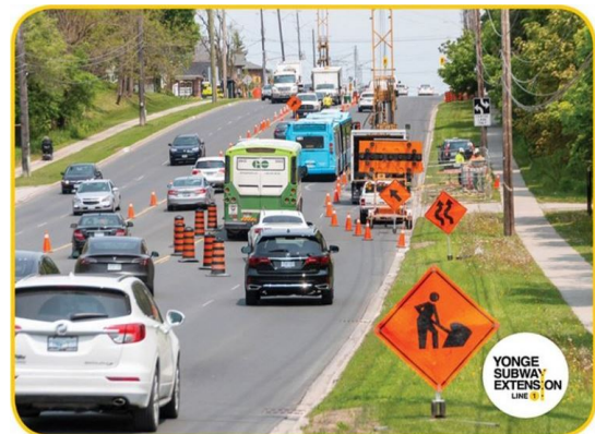
Geotechnical work underway on Yonge St.
