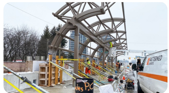
Steel vivastation canopy structure in place
