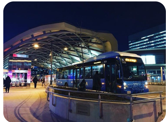
VMC rapidway station, connecting to TTC subway and SmartVMC Bus Terminal
