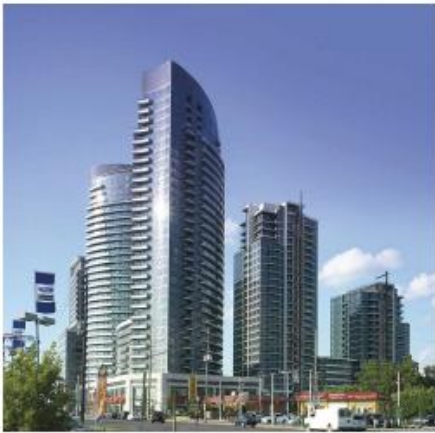
Figure 10 : Existing "World on Yonge" Development [north of Steeles Avenue]
