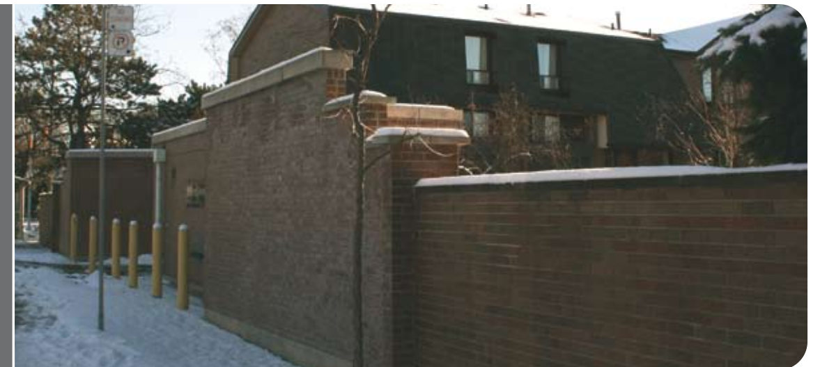
emergency exit building
