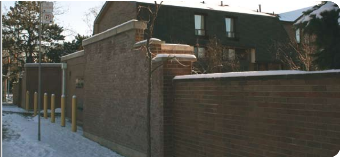
emergency exit building
