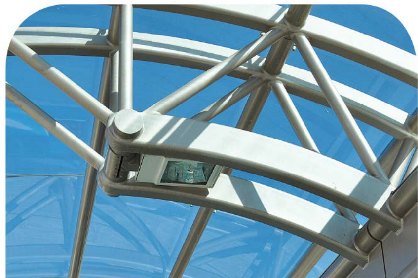
energy-efficient lighting throughout for greater safety and comfort
