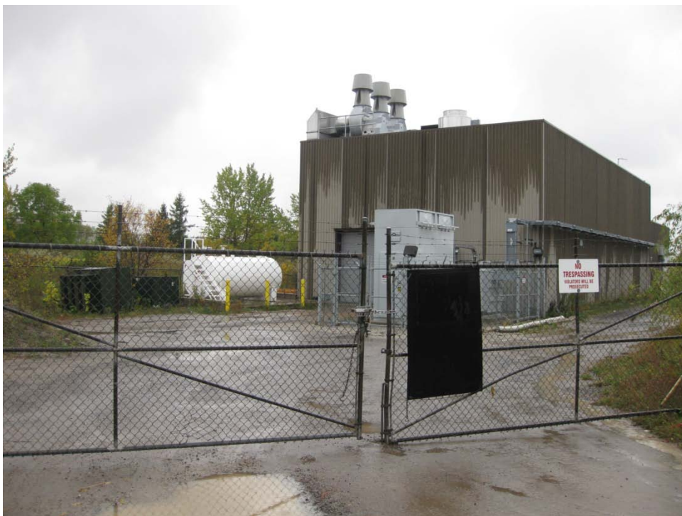
Photograph 20: View of the building and AST in the Black Creek Pumping Station adjacent to the southeast area of the Site.
