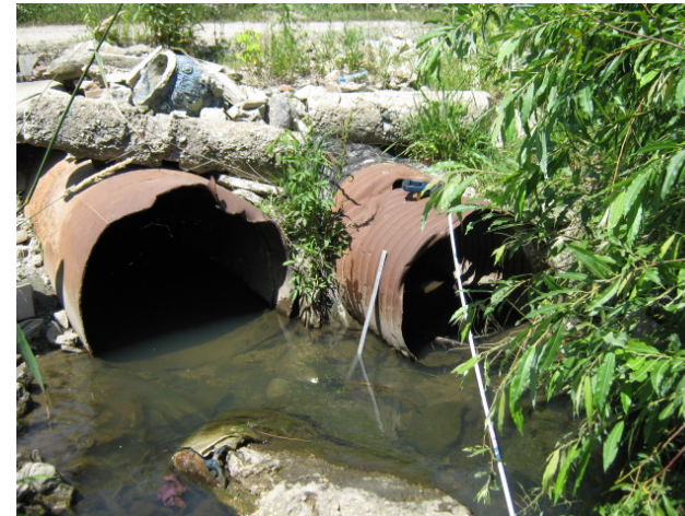
Plate 4. Double CSP culvert at top of Reach 2 (looking upstream)
