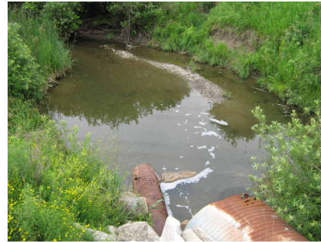
Plate 13. Double CSP culvert top of Reach 5 (looking downstream)
