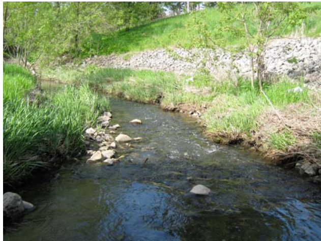
Plate 1 Riprap Reinforced Banks at Upstream section of Reach 1 below Jane Street culvert (looking downstream)
