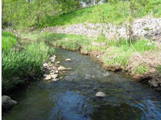
Figure 3-7 Riprap Reinforced Banks at Upstream section of Reach 1 (looking downstream)
