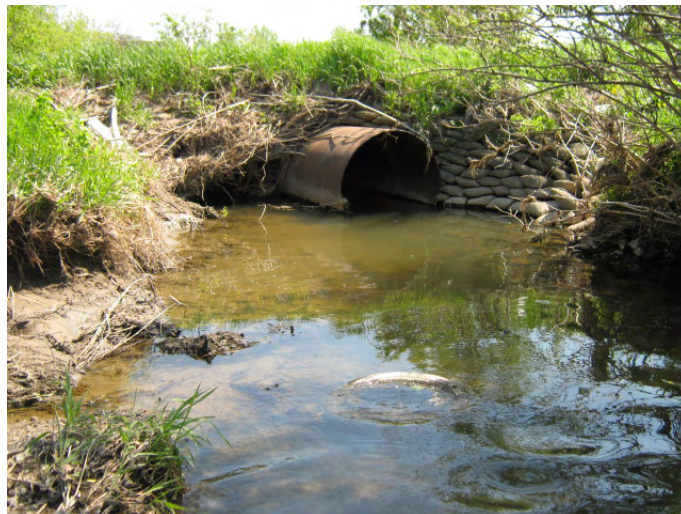
Figure 3-9 Crossing under HONI Access Road (looking downstream at CSP culverts)
