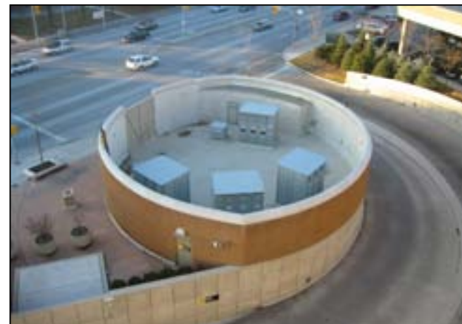
Aerial view of Don Mills Station substation showing substation enclosure and transformers
