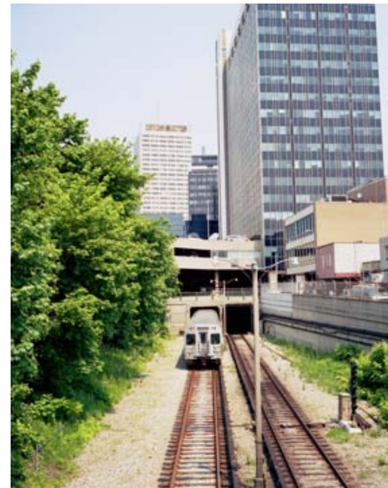
Figure 7-11: Open Cut section, Yonge Subway, South of Eglinton
