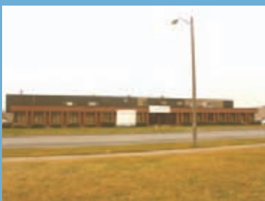
Steeprock Drive - large warehouse
