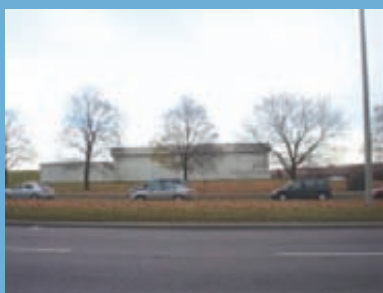
Keele Pumping Station
