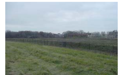
Plate 6: View of preferred alignment from Sheppard Avenue across field and connecting to Keele Street (in the distance); area will be tunneled.
