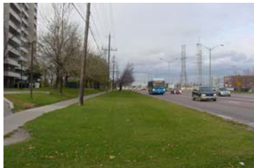
Plate 9: Looking north along Keele Street section of preferred alignment from proposed Finch West Station site; view of proposed pedestrian entrance.
