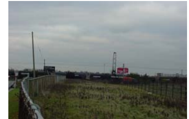
Plate 4: Looking east along Sheppard Avenue at proposed Downsview Park Station site beside railway tracks; cut and cover construction.
