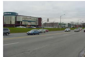
Plate 3: Looking northwest from Dufferin Street along preferred alignment that will run beneath buildings
