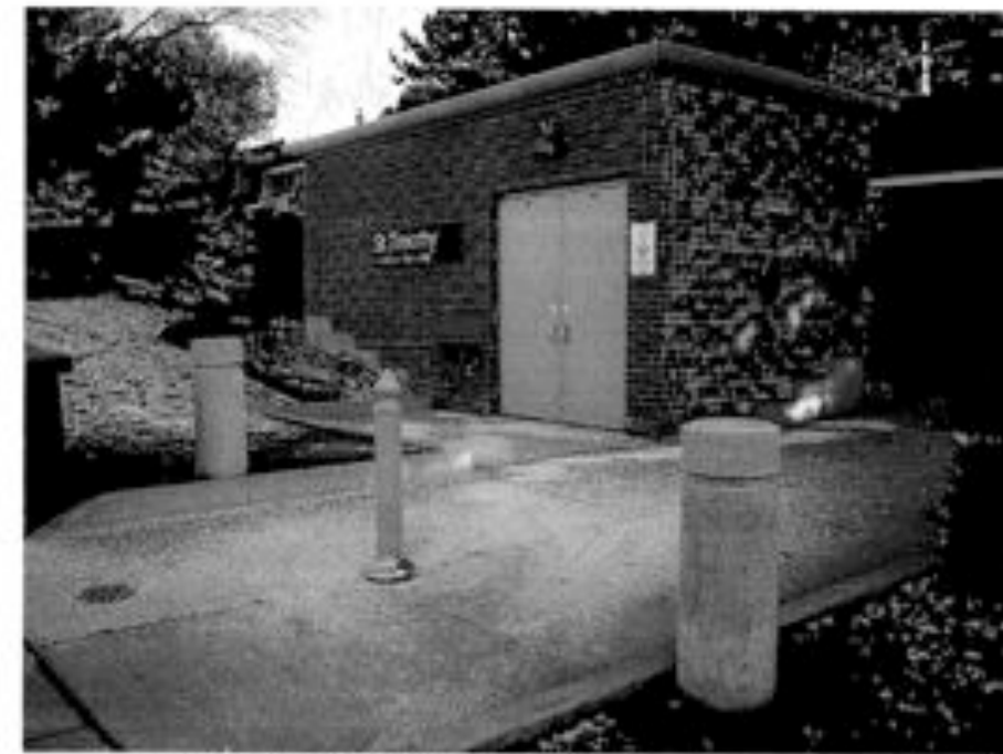
Sheppard Avenue East, west of Don Mills Road
