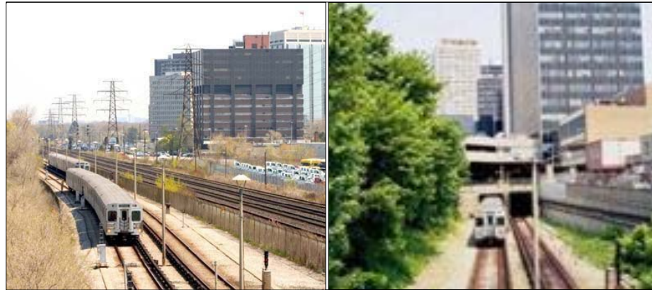
(Bloor-Danforth Subway at Kipling) (Yonge Subway at Eglinton) Open Cut
