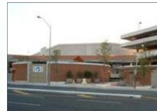
Electrical Substation (Don Mills Station)
