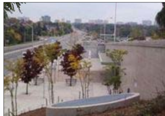
Ventilation Structure (Leslie Station)
