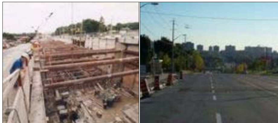
(Bessarion Station) (Sheppard Avenue) Cut – and – Cover
