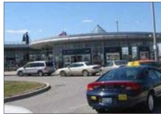
Passenger Pick-Up/Drop-off (Downsview Station)
