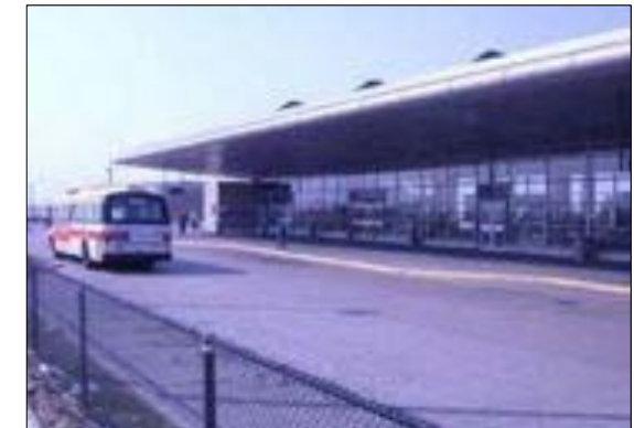
Bus Terminal (surface) (Downsview Station)
