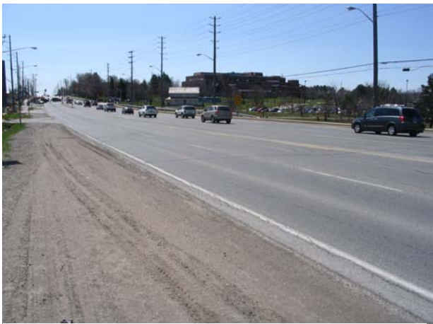
Plate 9: View to south along Yonge Street, from Gladman Avenue
