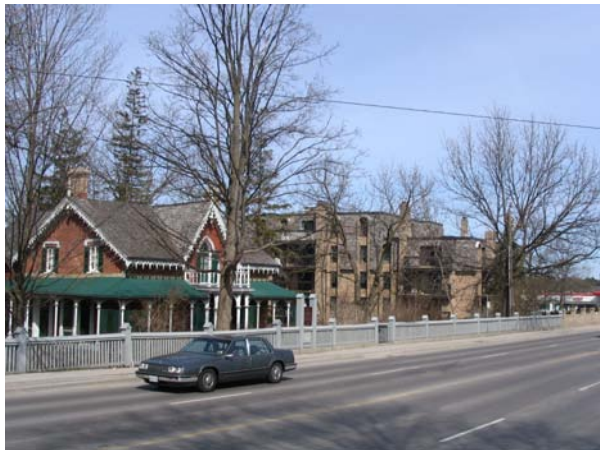
Plate 12: View to northwest from northeast corner of Yonge Street and Maple Street looking at mid-late 19 th century farm house on land below grade.
