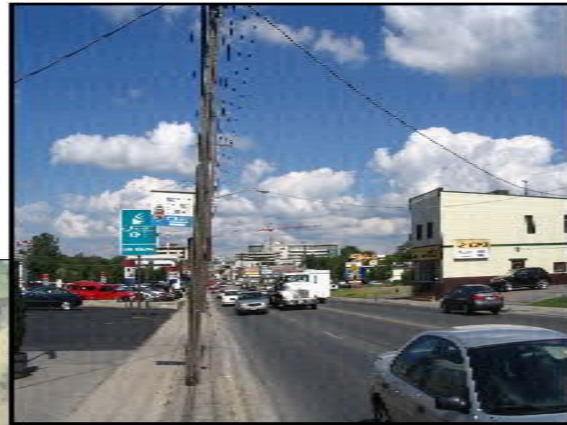
Plate 48: Looking east along Davis Drive from Main Street at commercial development on both sides of ROW.
