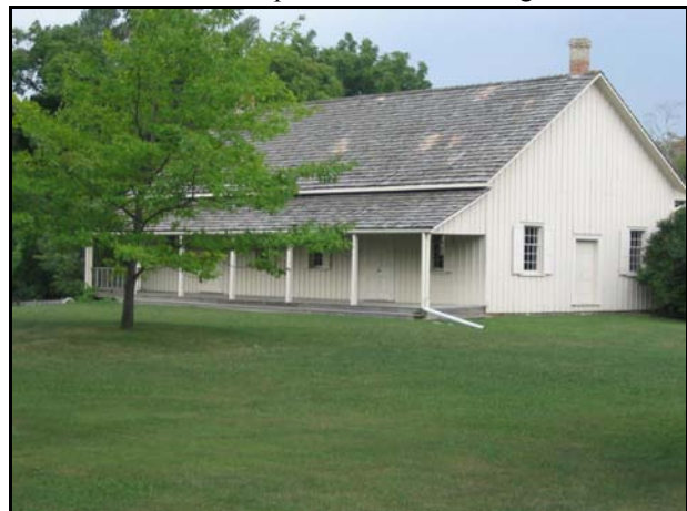
Plate 4: View to northwest. Quaker meeting house (1812) situated on the west side of Yonge Street, south of Eagle Street intersection.
