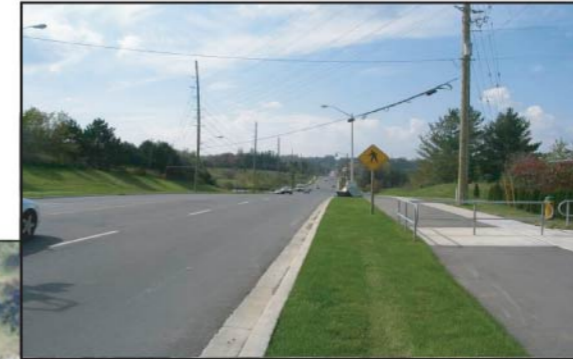
Plate 28: View to the west-southwest along St. Johns Sideroad towards Yonge Street at top of second ridge in distance. Cut and filled roadbed beyond.
