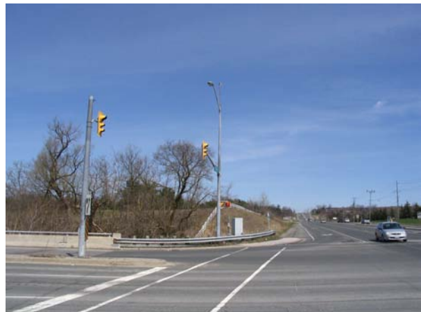
Plate 17: View from southwest corner of Yonge Street and St. John's Sideroad showing higher ground to the north.
