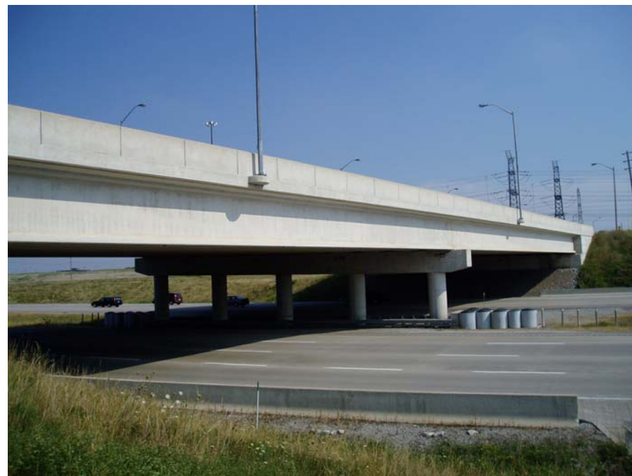
Figure 9-10 Warden Avenue Crossing Highway 407
