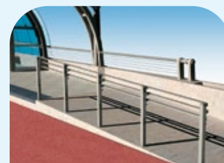
gently sloping ramp provides easy wheelchair, motorized scooter and stroller access
